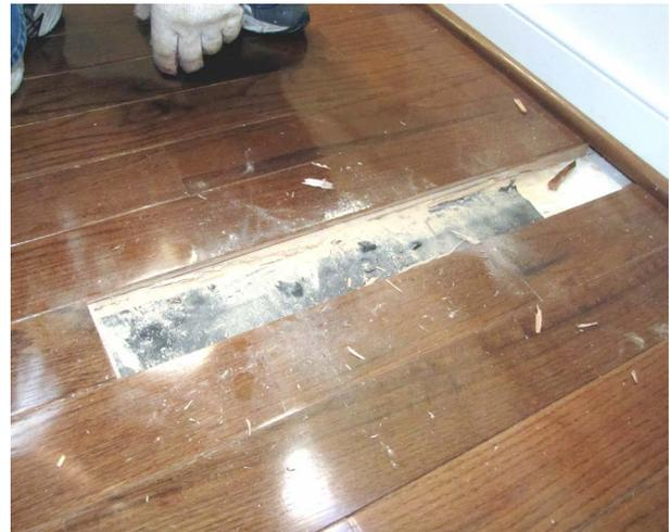
Replacing a section of powderpost beetle-infested and damaged wood is a nonchemical control option (Pinto)
